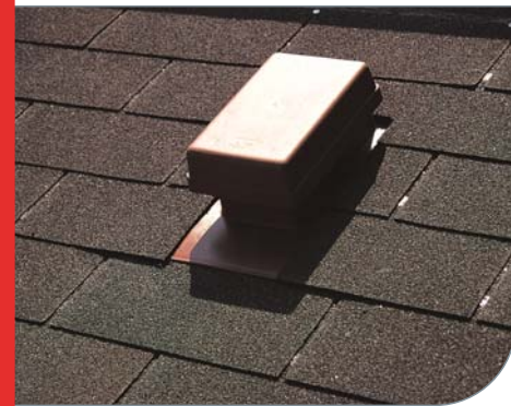
3 3 Special ventilation element
